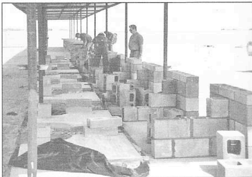
Figure 5. Pedestals made of concrete blocks. Mooreland, OK.
