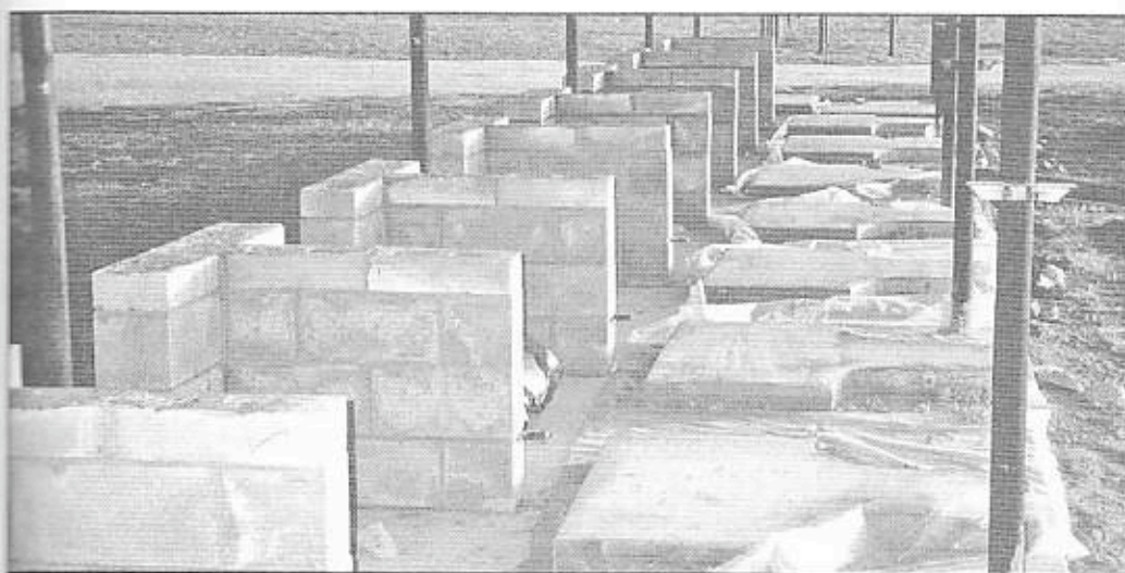
Figure 7. Tops poured behind the pedestals on which they will rest.
